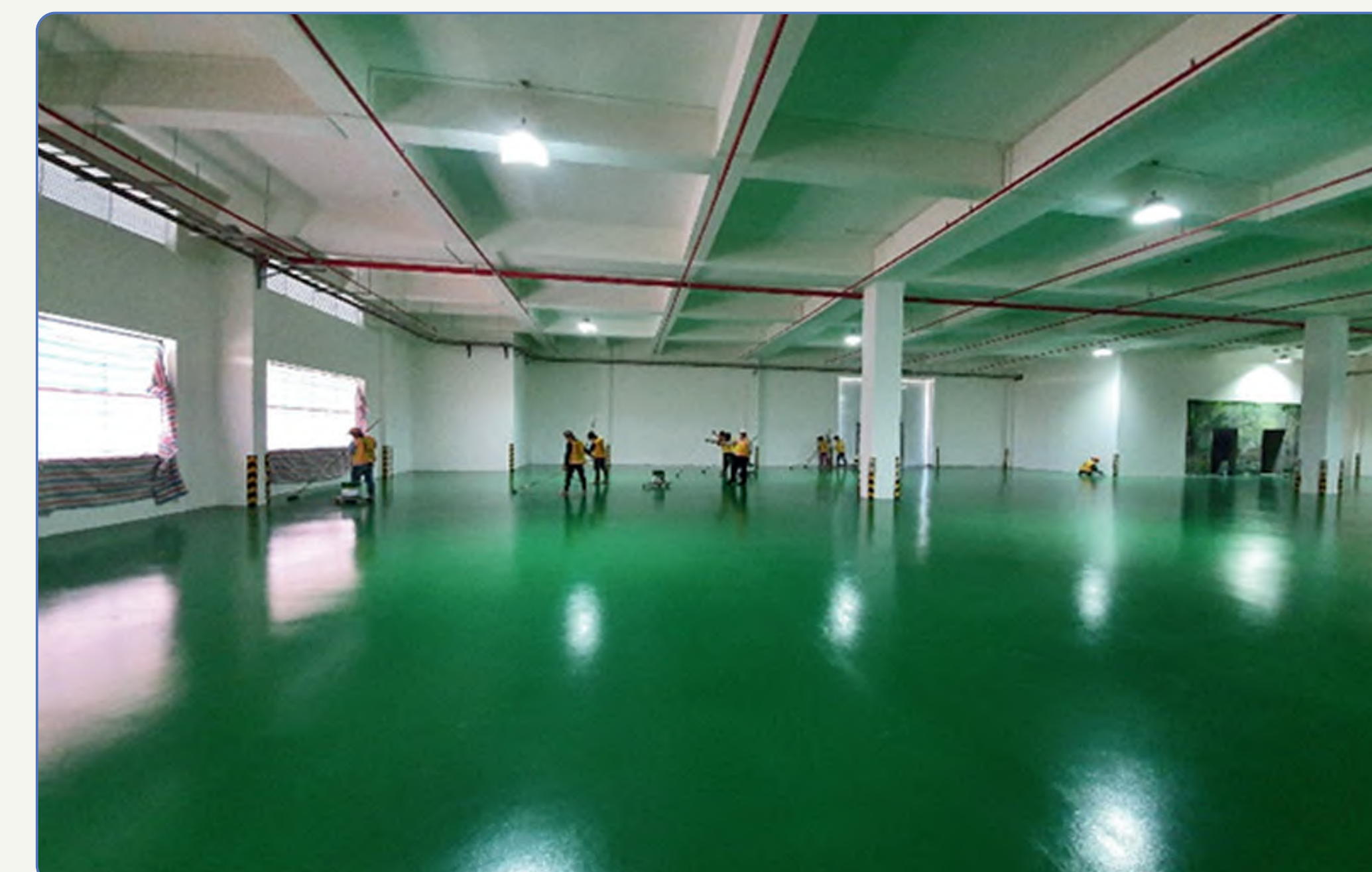
Epoxy Floor Application
