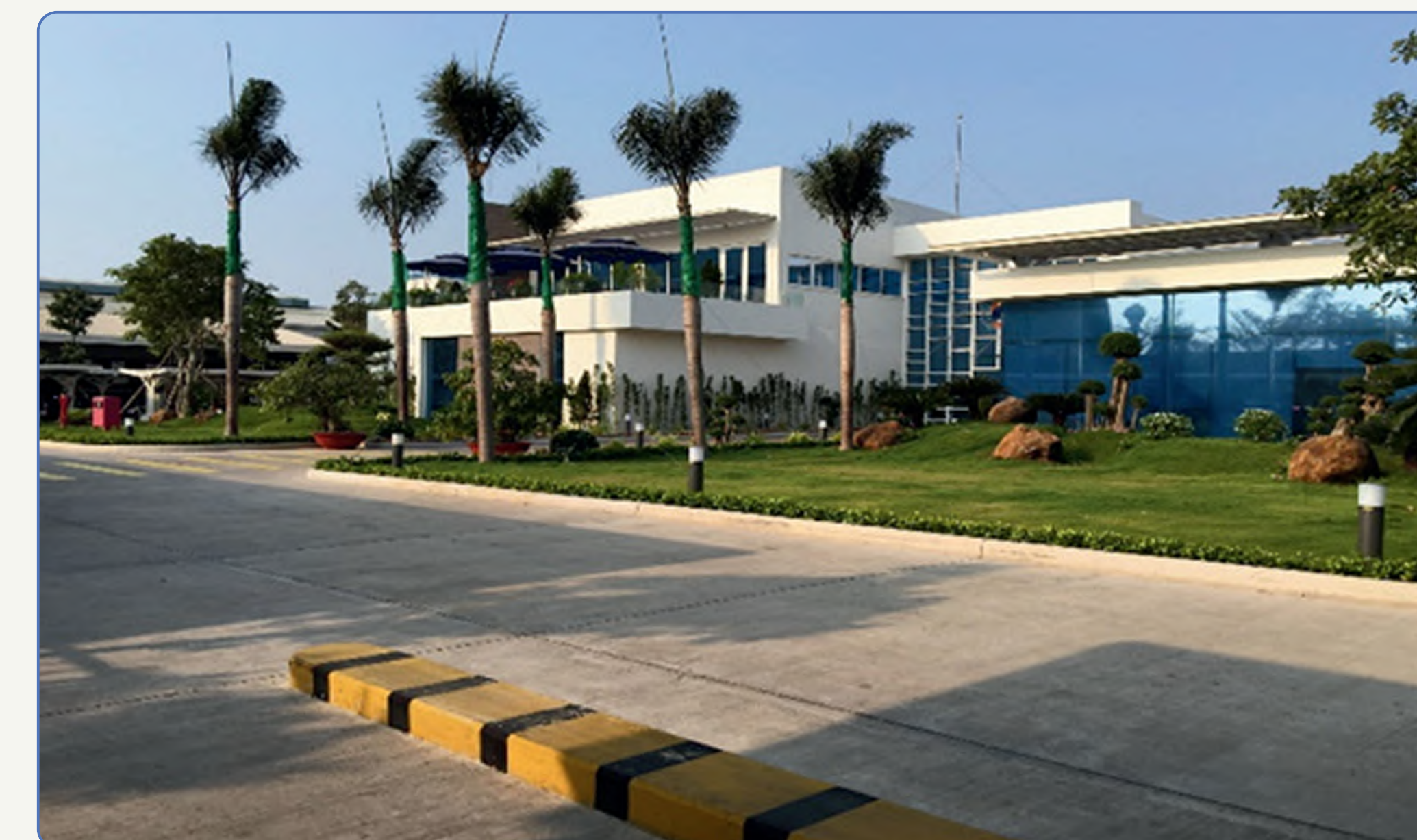
Concrete Road Pavement
