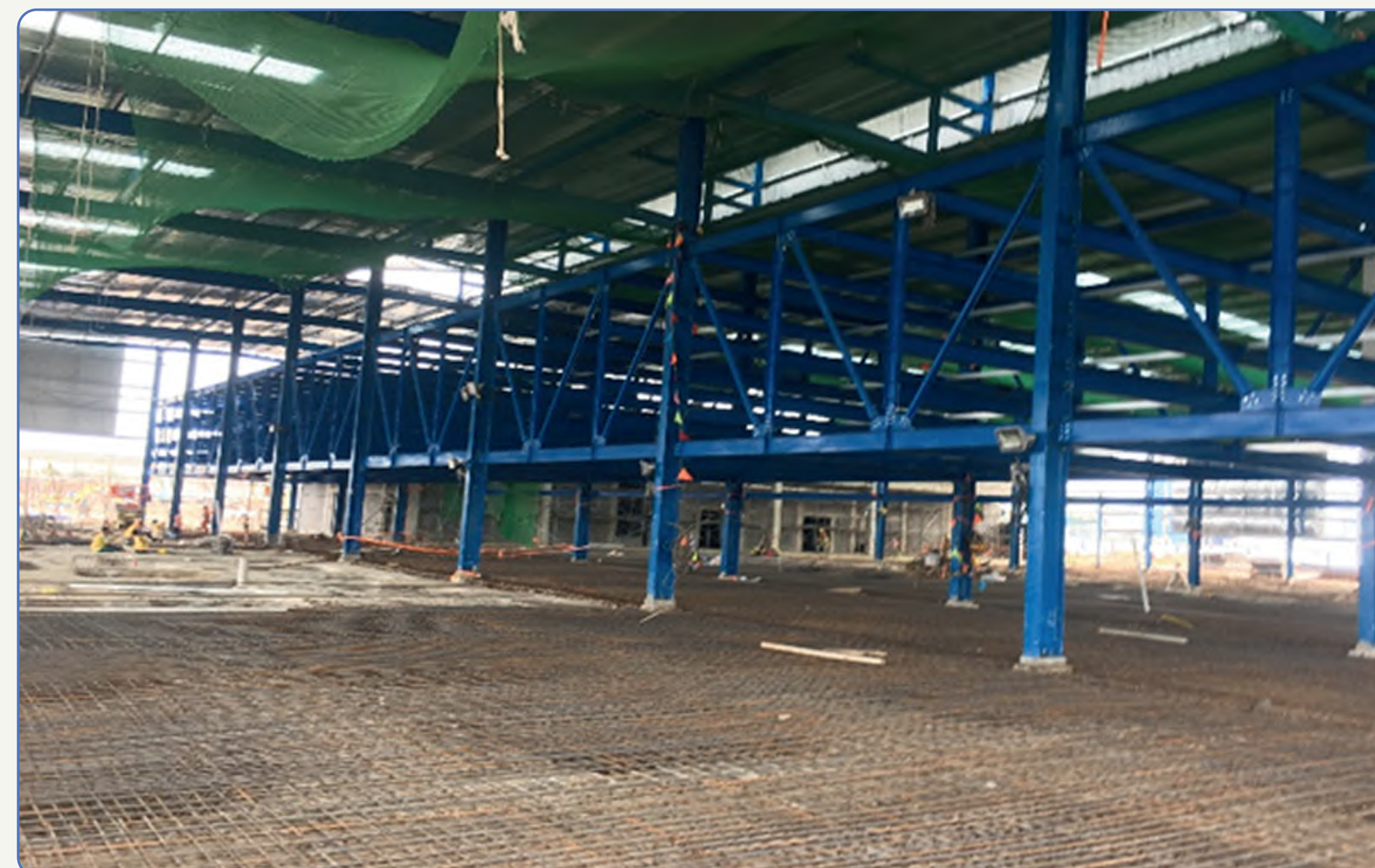
Ground Slab Rebar Installation
