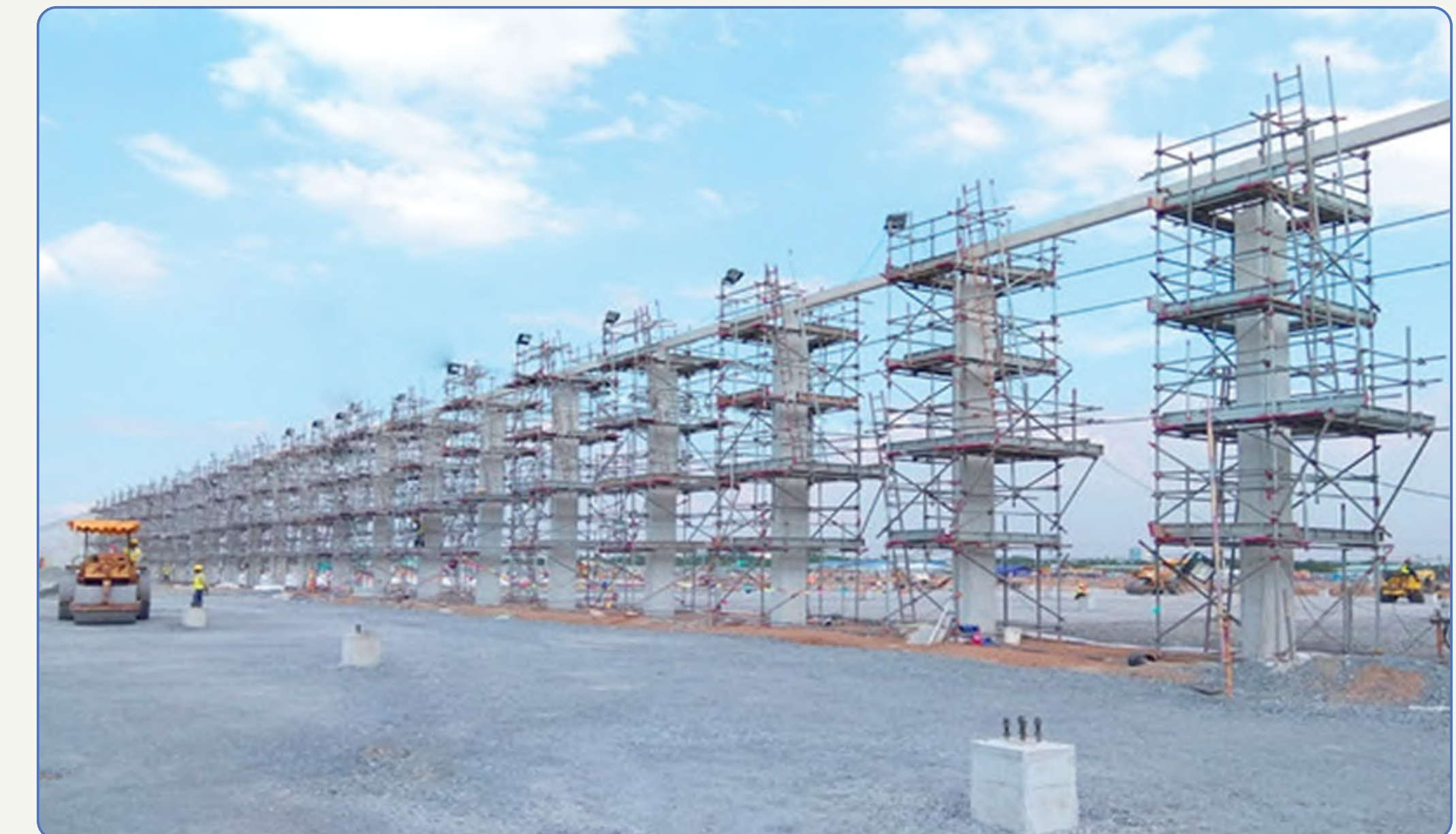
High-column Concrete Casting
