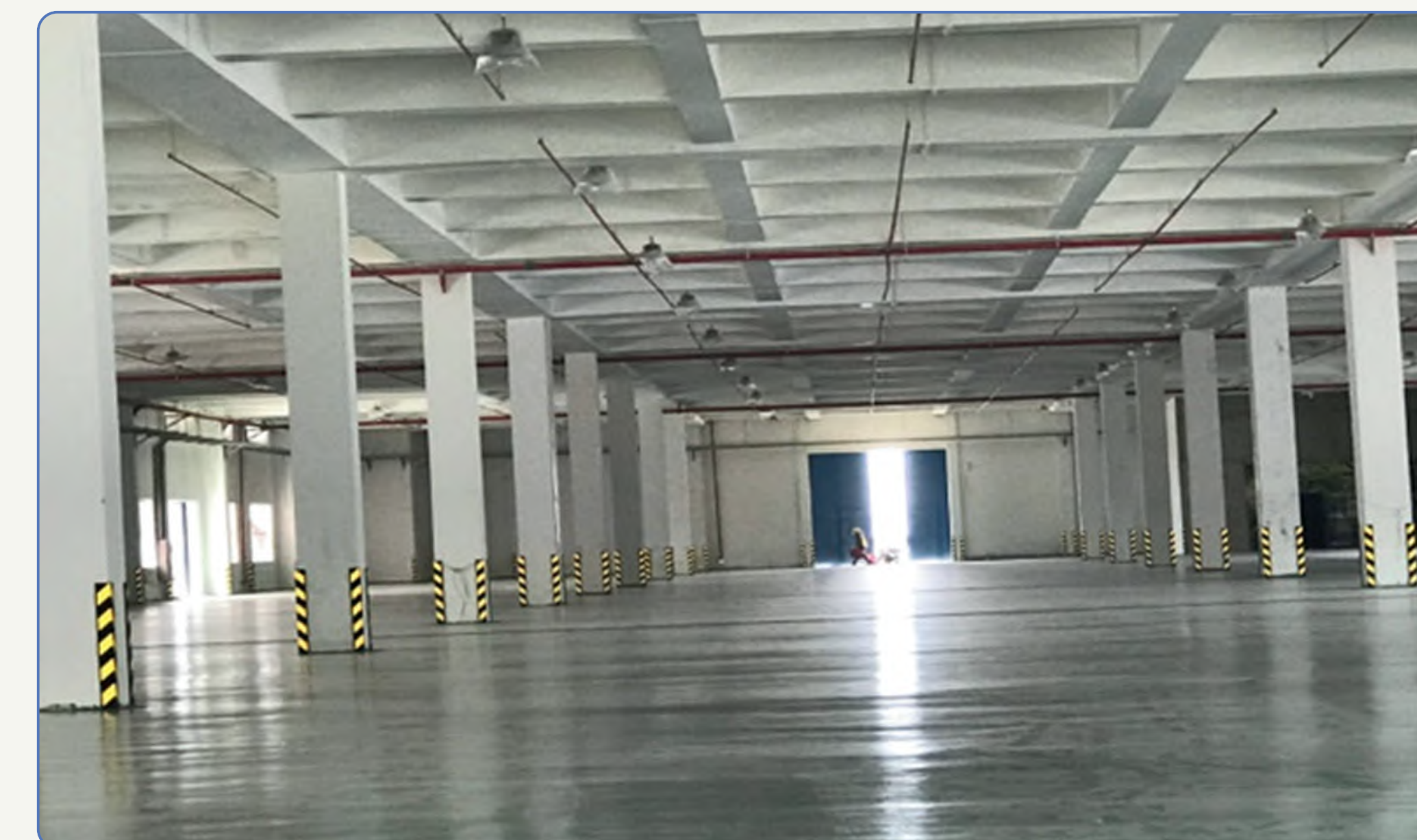
Inside Factory Finishing
