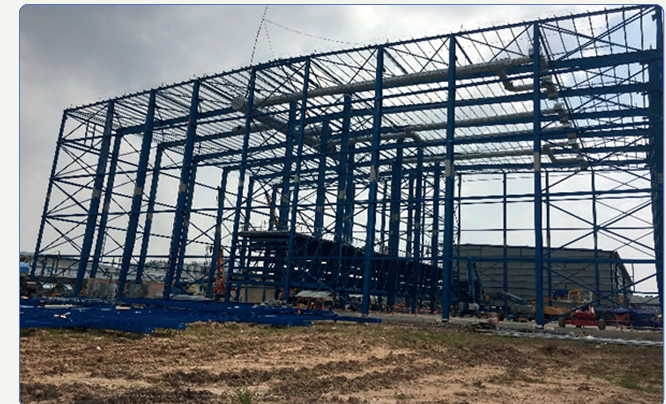
Steel Structure Erection
