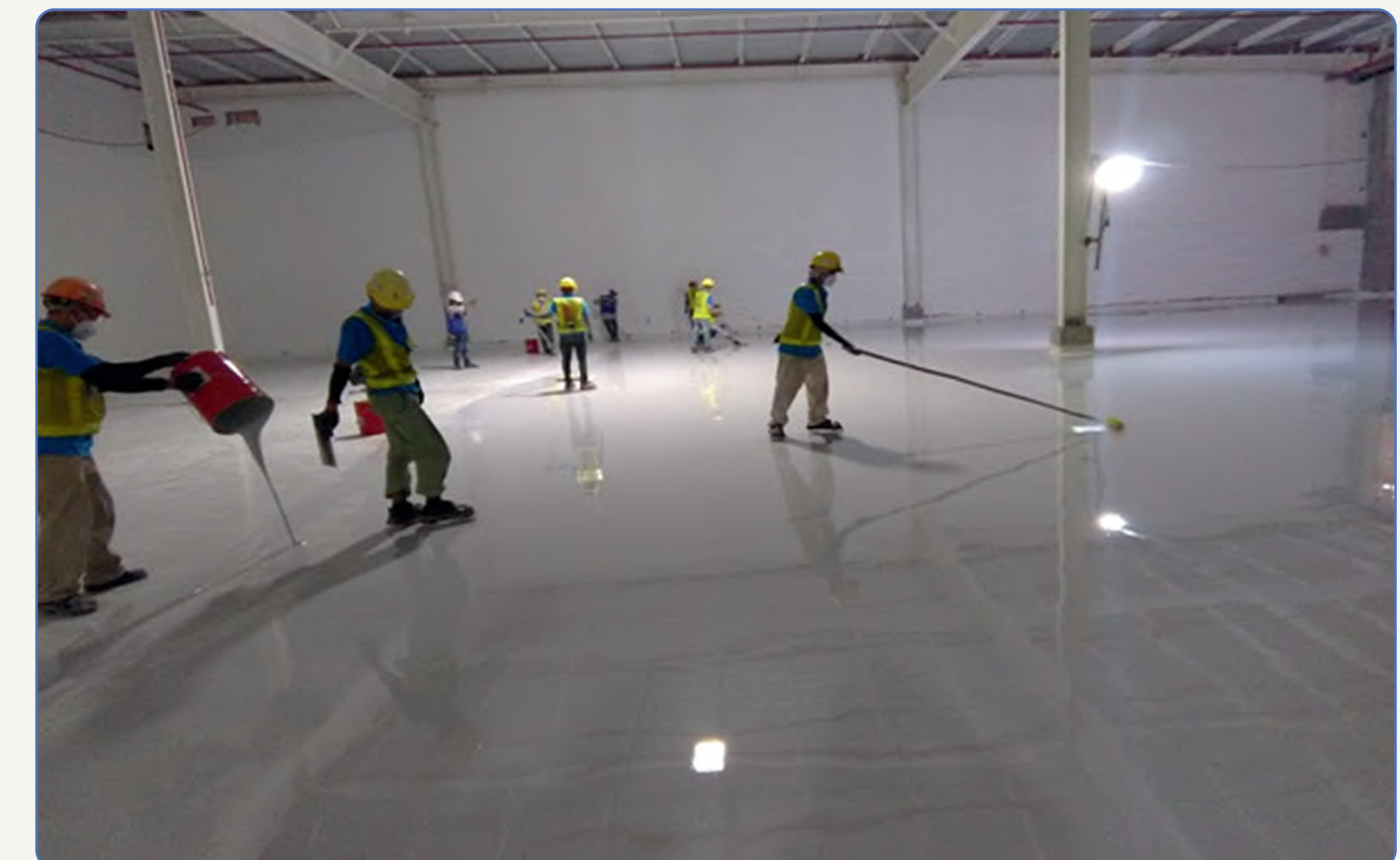
Epoxy Floor Application
