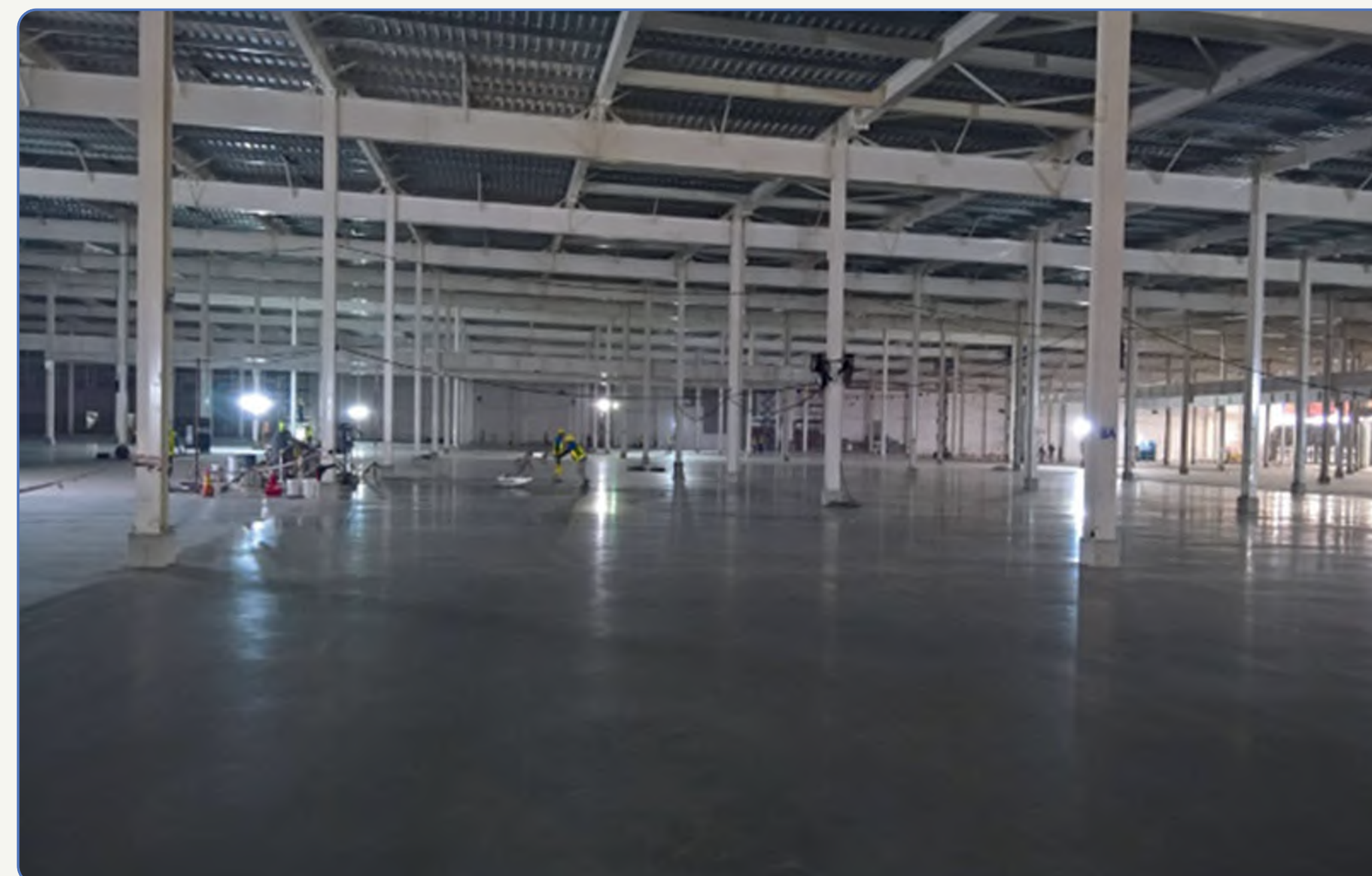
Floor Hardener Application
