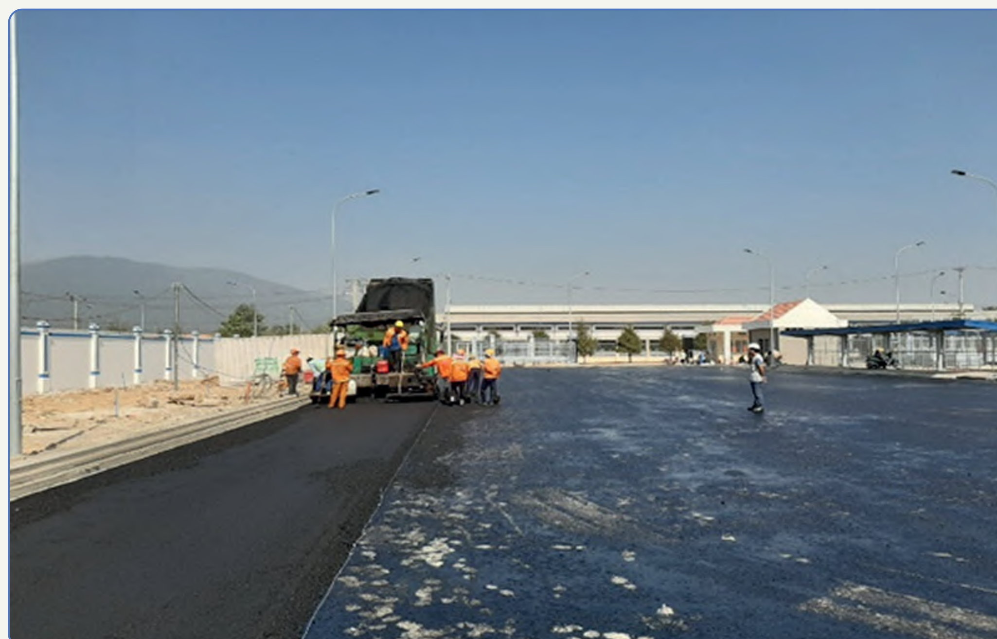
Asphalt Road Pavement
